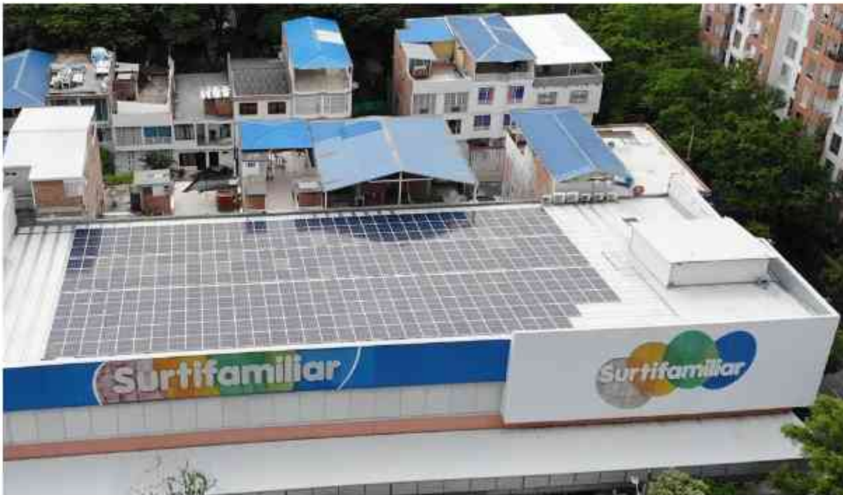
Surtifamiliar, 731,68 Kwp - Cali Colombia
