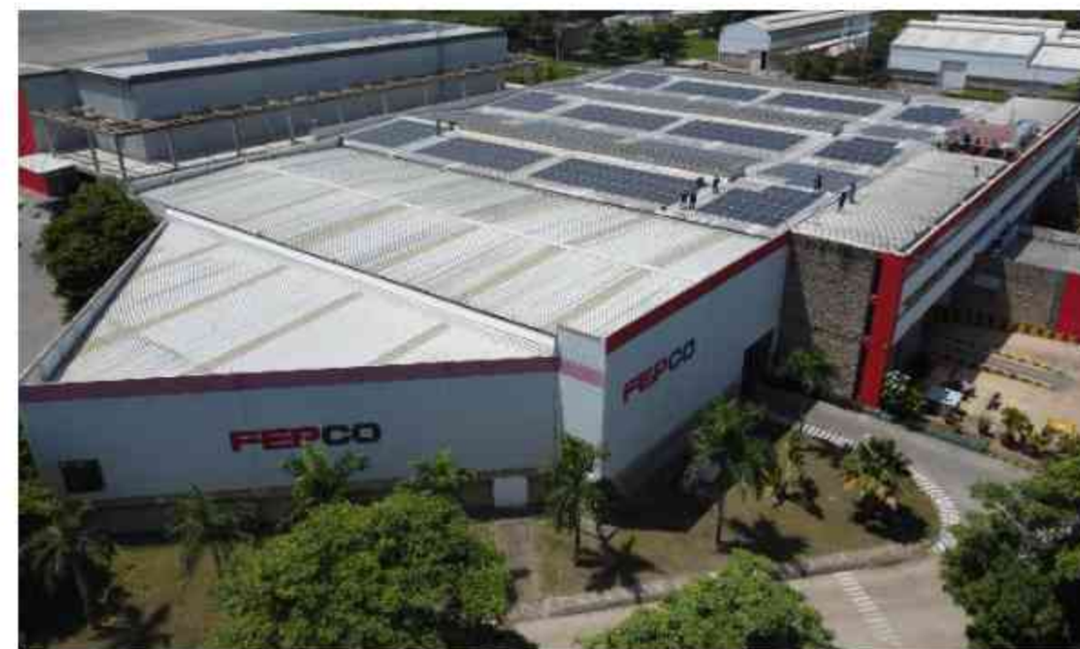
Fepco, 550 Kwp - Cartagena Bolivar
