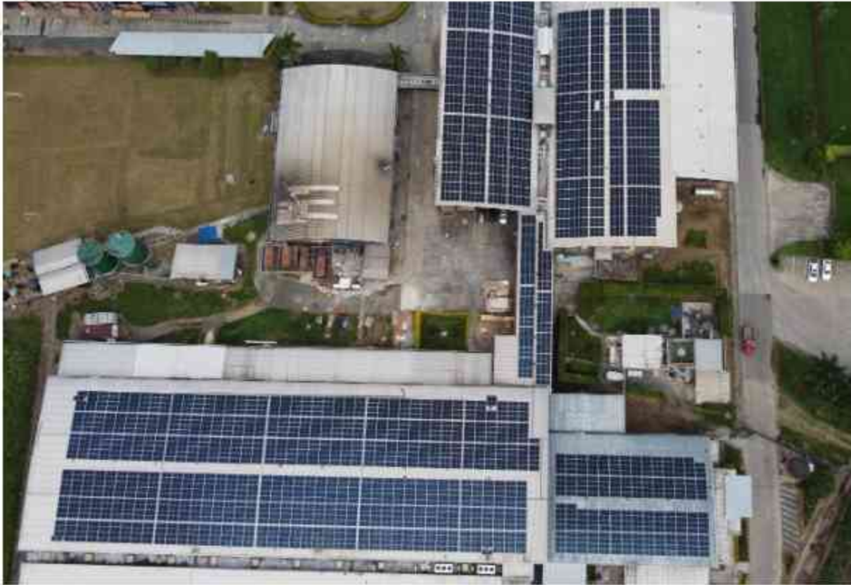
Alival, 1455 paneles - 1058 Kwp - Caloto Cauca
